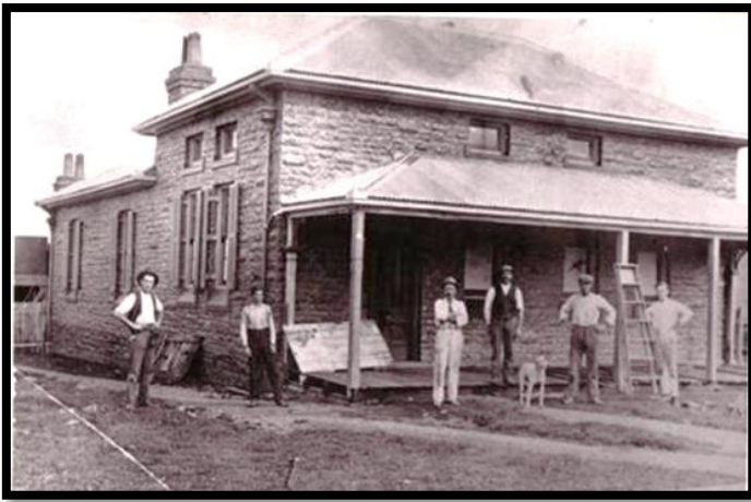
Kiandra Courthouse and police station, c. 1917.
